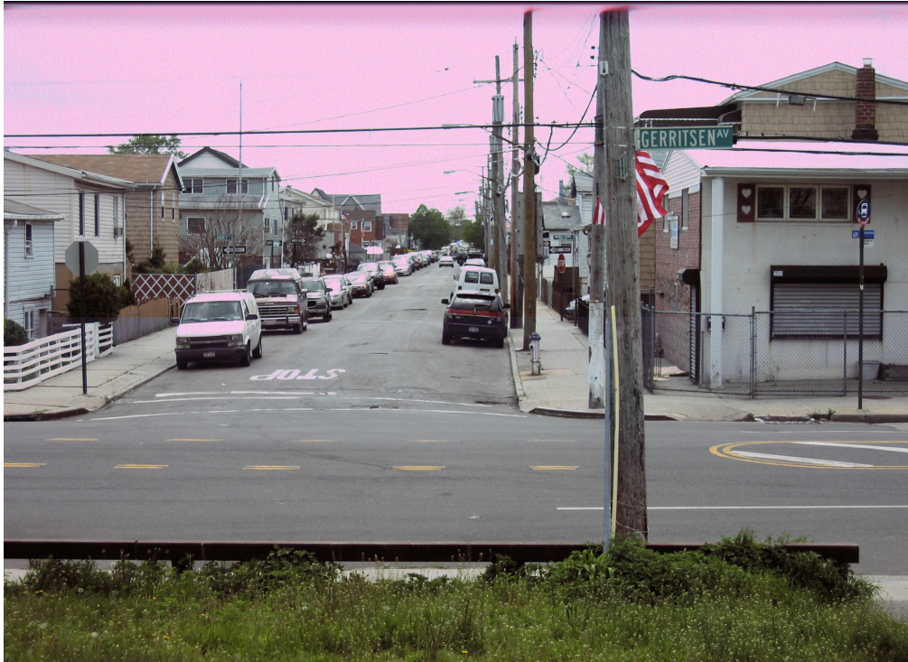
Image 4.1 Housing off of Gerritsen Avenue in Gerritsen Beach Brooklyn. Photo Van Hooreweghe
