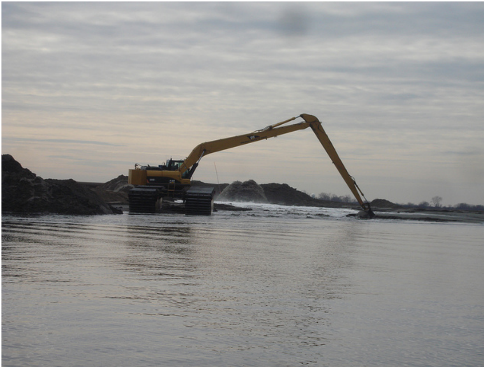
Image 2.6 A backhoe moves sand for a Jamaica Bay restoration project. Photo Jamaica Bay Eco-Watchers
