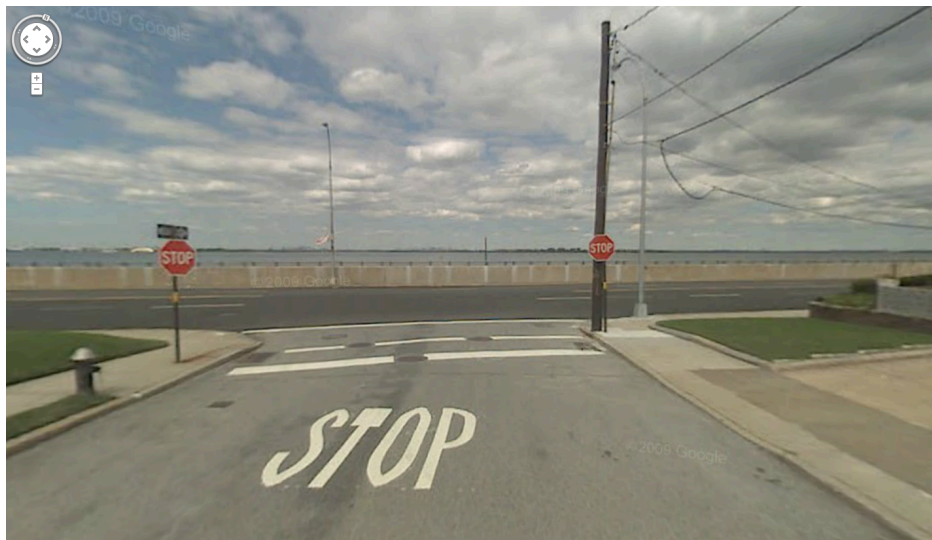
Image 4.36 View of the Seawall along Beach Channel Drive and Beach 132 nd St. Photo Google Street View
