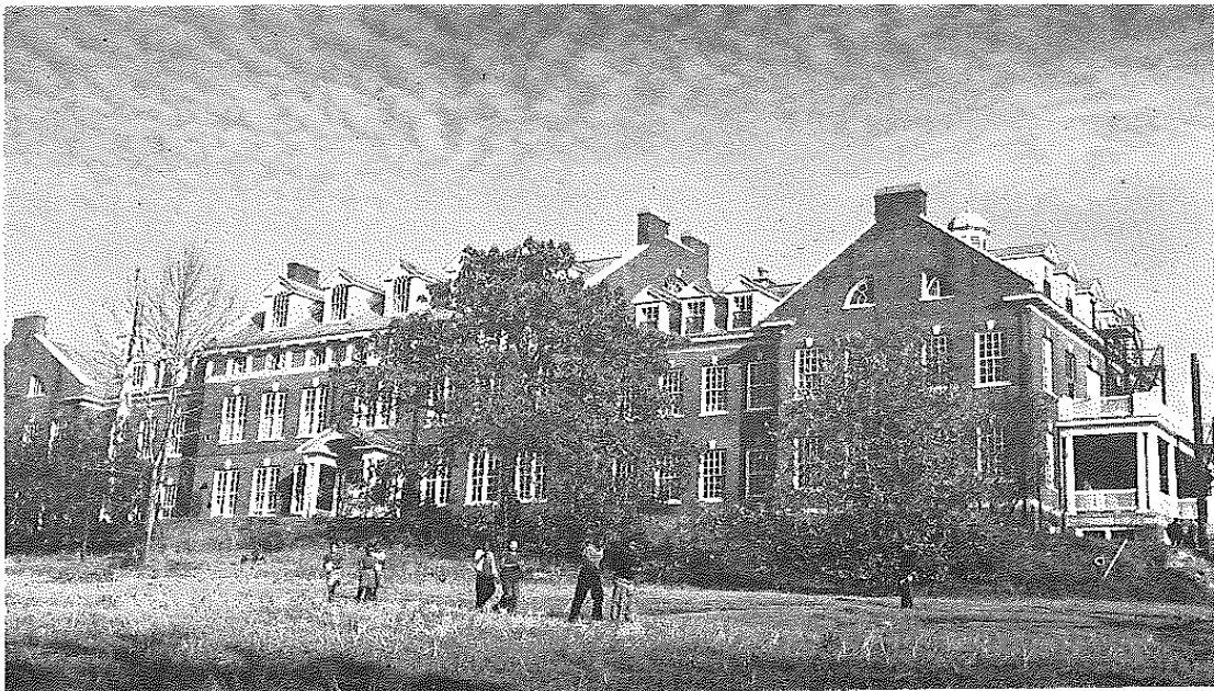
The main building of the Colored Orphans' Asylum at Riverdale was occupied from 1907 to 1946. It housed the school, administrative offices, the hospital, rooms for the staff, and dormitories for some of the children.
