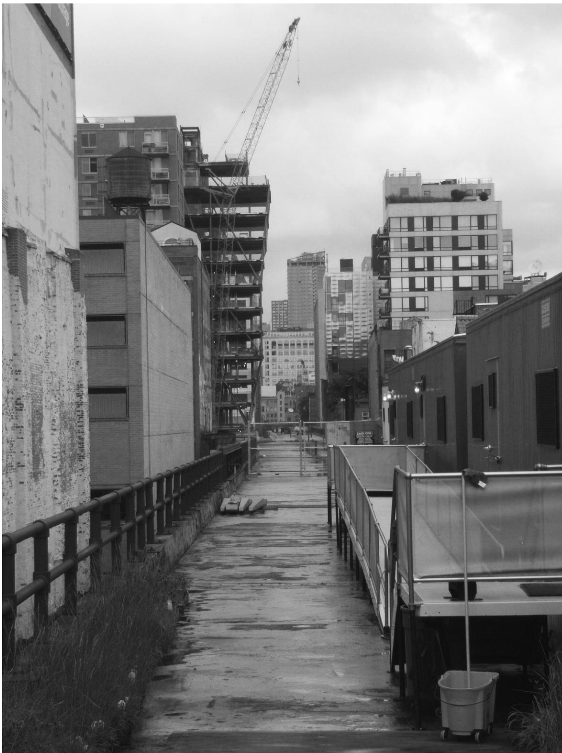
Figure 11: New buildings under construction along the unfinished northern section of the High Line. Building of the elevated park has “catalyzed” development by helping enhance real-estate values in formerly industrial areas on Manhattan’s Far West Side (Photo by the author, Aug. 1, 2009).
