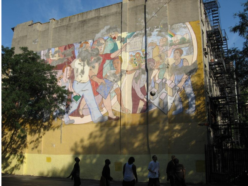
“Against Domestic Colonialism” in its state of disrepair
