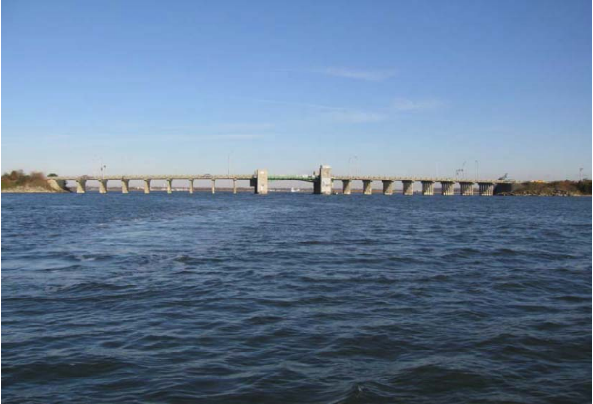
Figure 32: North fascia of Loop Parkway over Long Creek (Boswell 2009)
