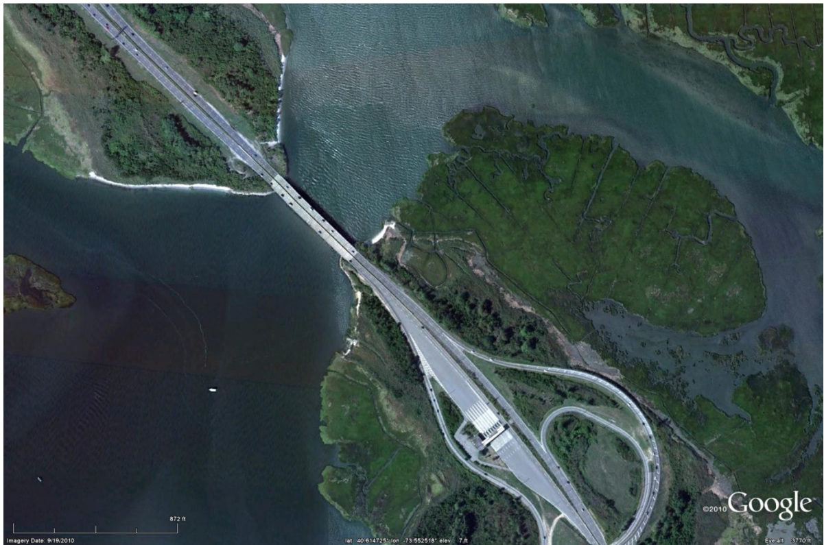
Figure 45: Aerial image of Meadowbrook Parkway over Fundy Channel (Google 2010)
