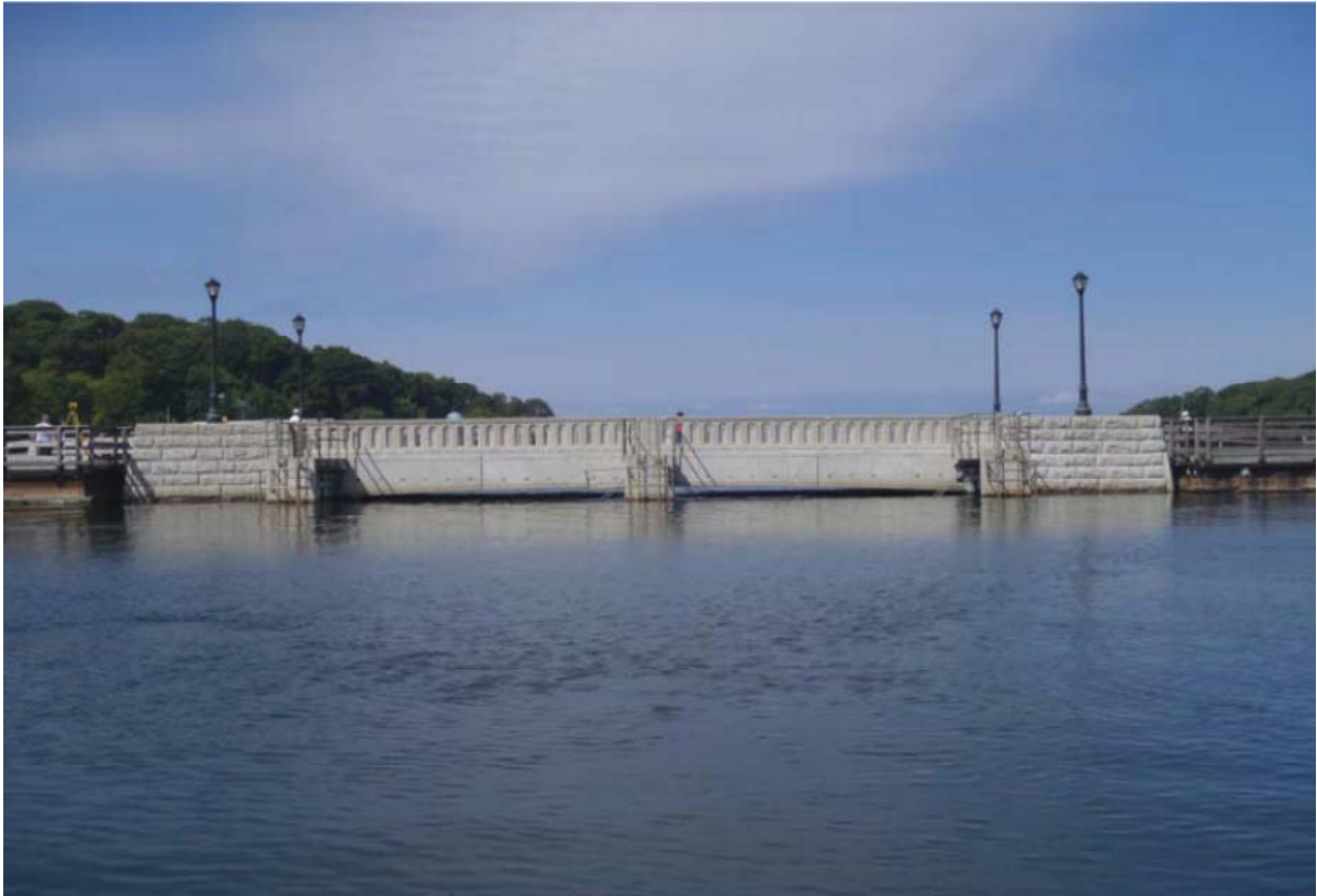
Figure 25: South fascia elevation of Mill Dam Road over Centerport Harbor (Boswell, 2010)
