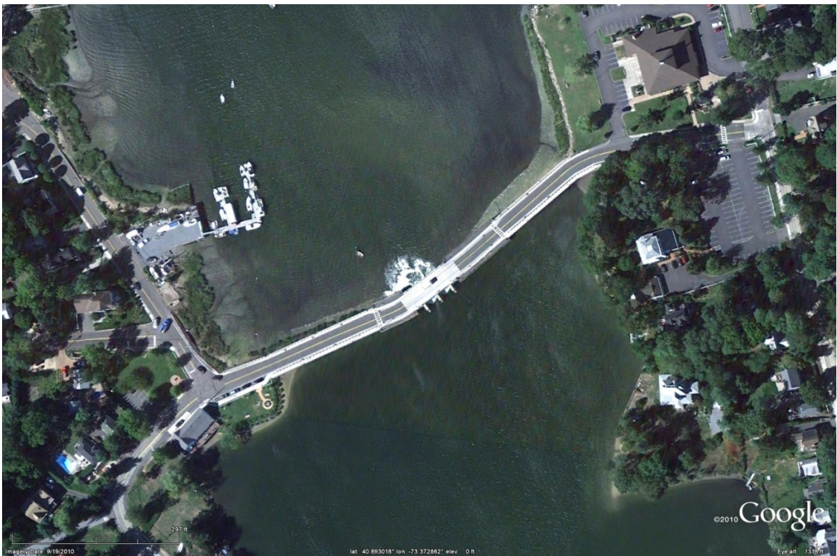
Figure 24: Aerial image of Mill Dam Road over Centerport Harbor (Google 2010)
