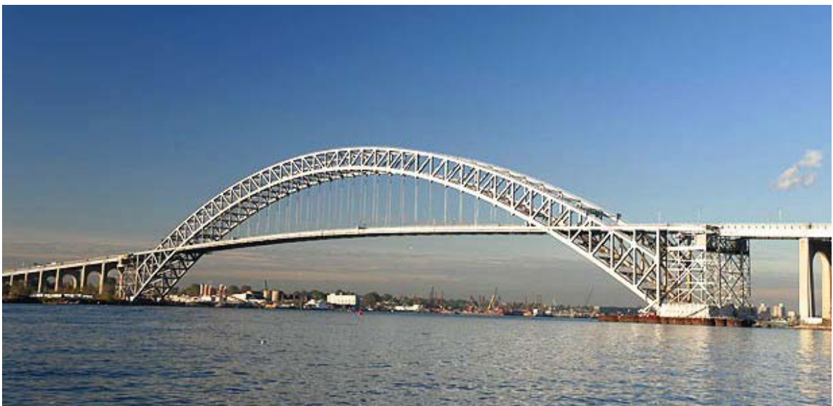
Figure 49: Bayonne Bridge looking East over the Kill Van Kull (PANYNJ, 2011)
