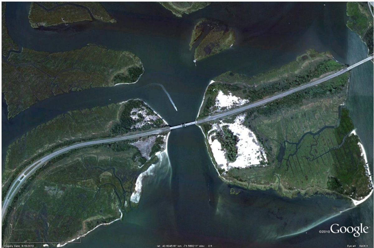
Figure 31: Aerial image of Loop Parkway over Long Creek (Google 2010)
