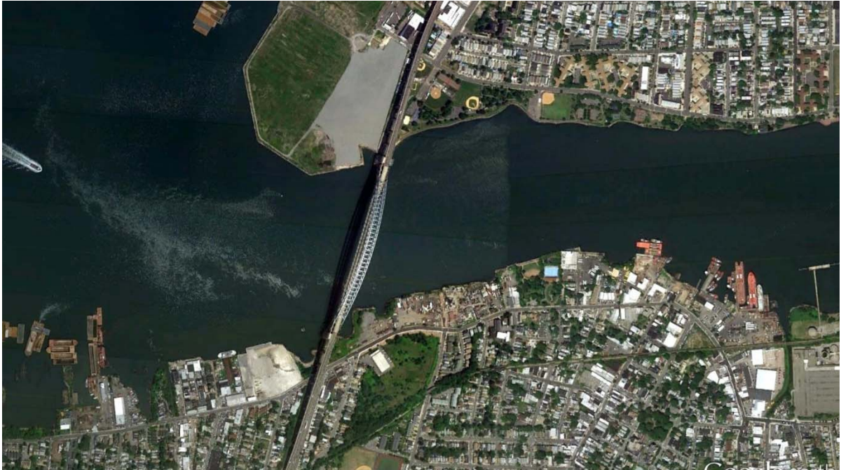
Figure 48: Aerial image of Bayonne Bridge over Kill Van Kull (Google, 2010)
