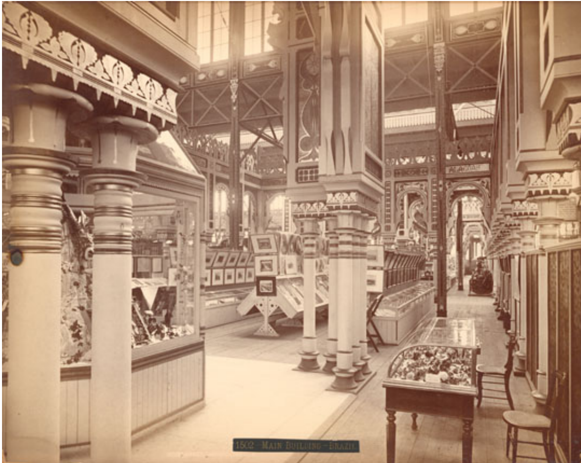
Figure 11: Centennial Photographic Company, "Brazilian Court in Main Building," Architect Frank Furness, Free Library of Philadelphia, c021502. Photographs rarely had visitors in the frame, as exposure times of cameras rendered them blurry, thus contributing to an idealized, orderly vision of the fair. One must imagine a popular space like this rather cramped.
