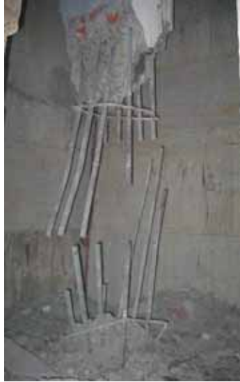
Figure 6.13: Severance of longitudinal rebars during a test by Matthews et al. (2007).
