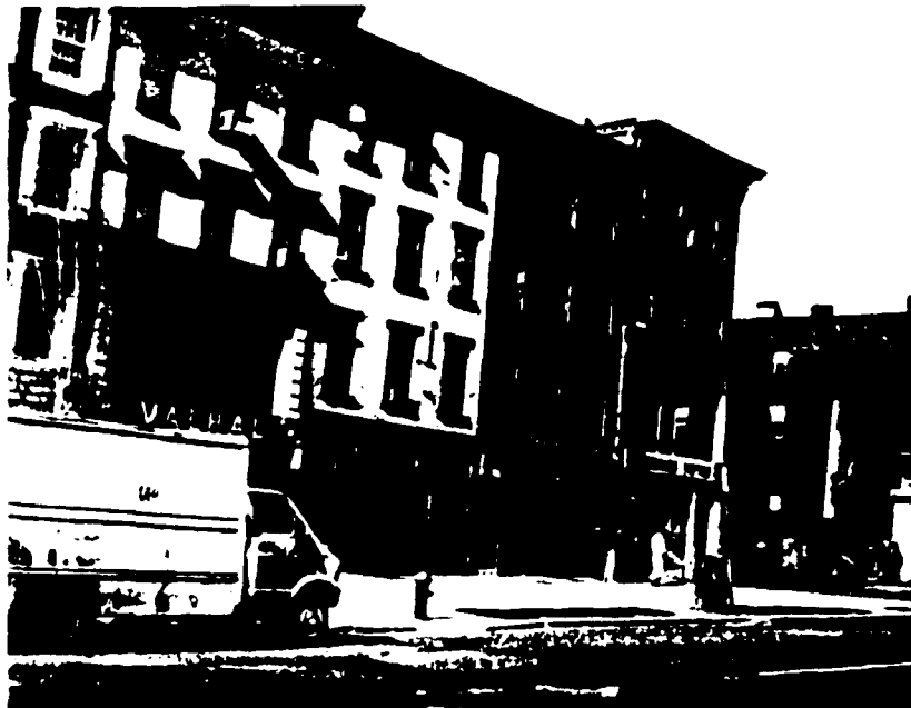
Fulton Street, awaiting restoration.
