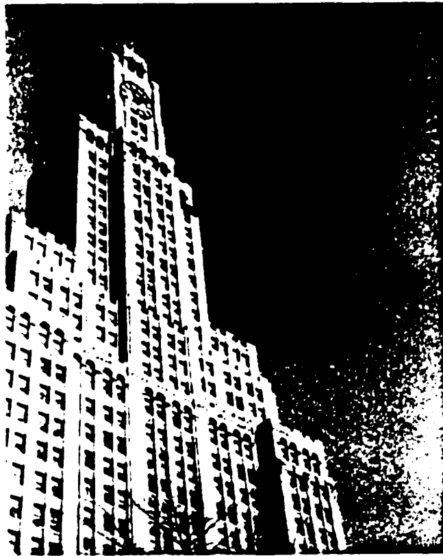
Williamsburg Savings Bank, Ashland Place and Hanson Place
