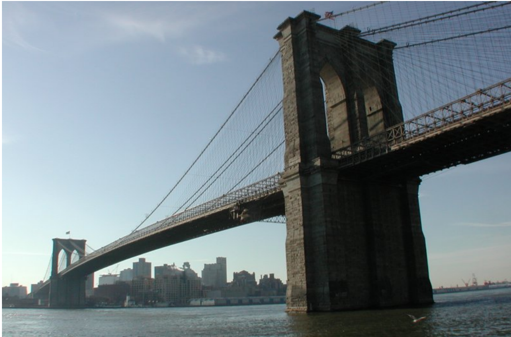
Figure 5.1: Unreinforced masonry tower of the Brooklyn Bridge as its most prominent features
