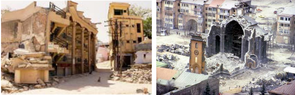
Figure 1.1: Collapse of masonry buildings and churches during the earthquake
