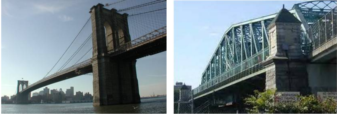
Figure 1.2: The Brooklyn Bridge with unreinforced masonry tower (left) and the 145th street Bridge in Manhattan with masonry piers (right)
