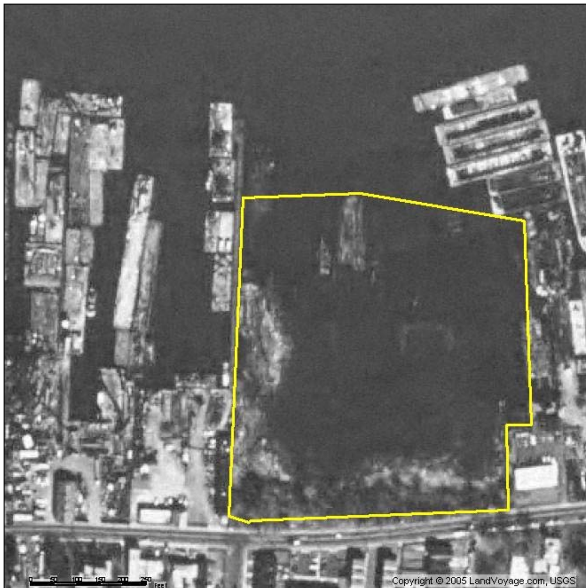
Figure A- 31: Site code KVKS2 – north of Richmond Terrace between Van Name and Van Pelt Avenues, Staten Island, NY (Richmond Co.)
