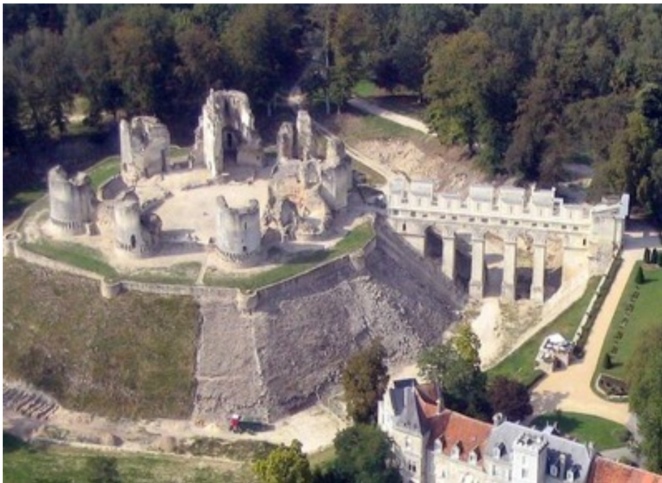
Fig. 22 Château de Fère-en-Tardenois, View from the South.
