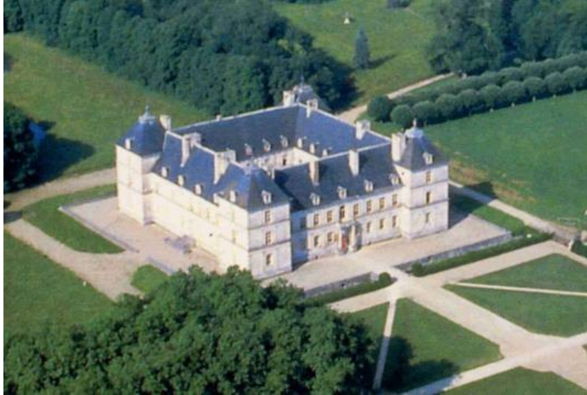
Fig. 3 Ancy-le-Franc, View of the Chateau from the Southwest.
