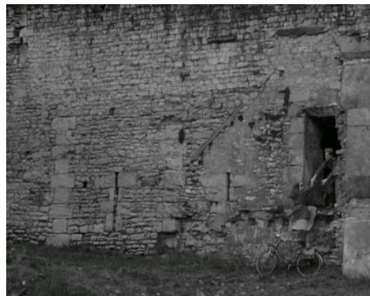
Figure 3.8 – An entrance in the village wall.
