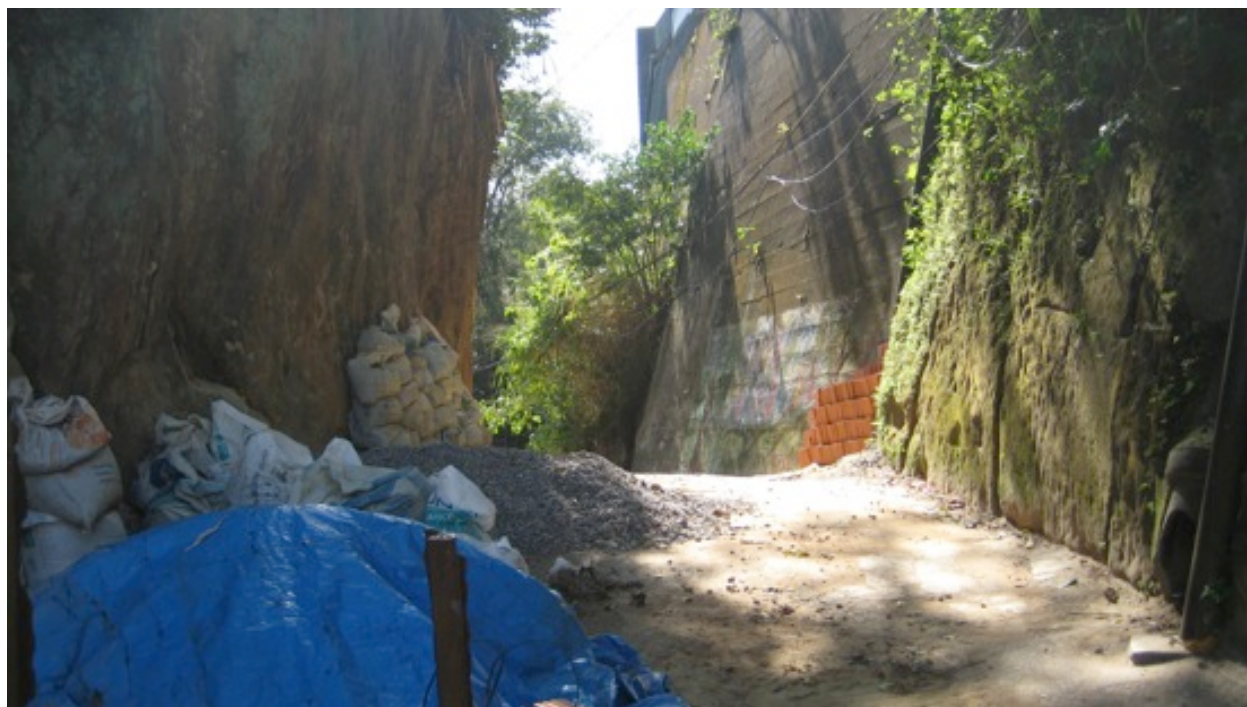
Figure 3 O túnel, upper entrance to Morro do Saqualé.
