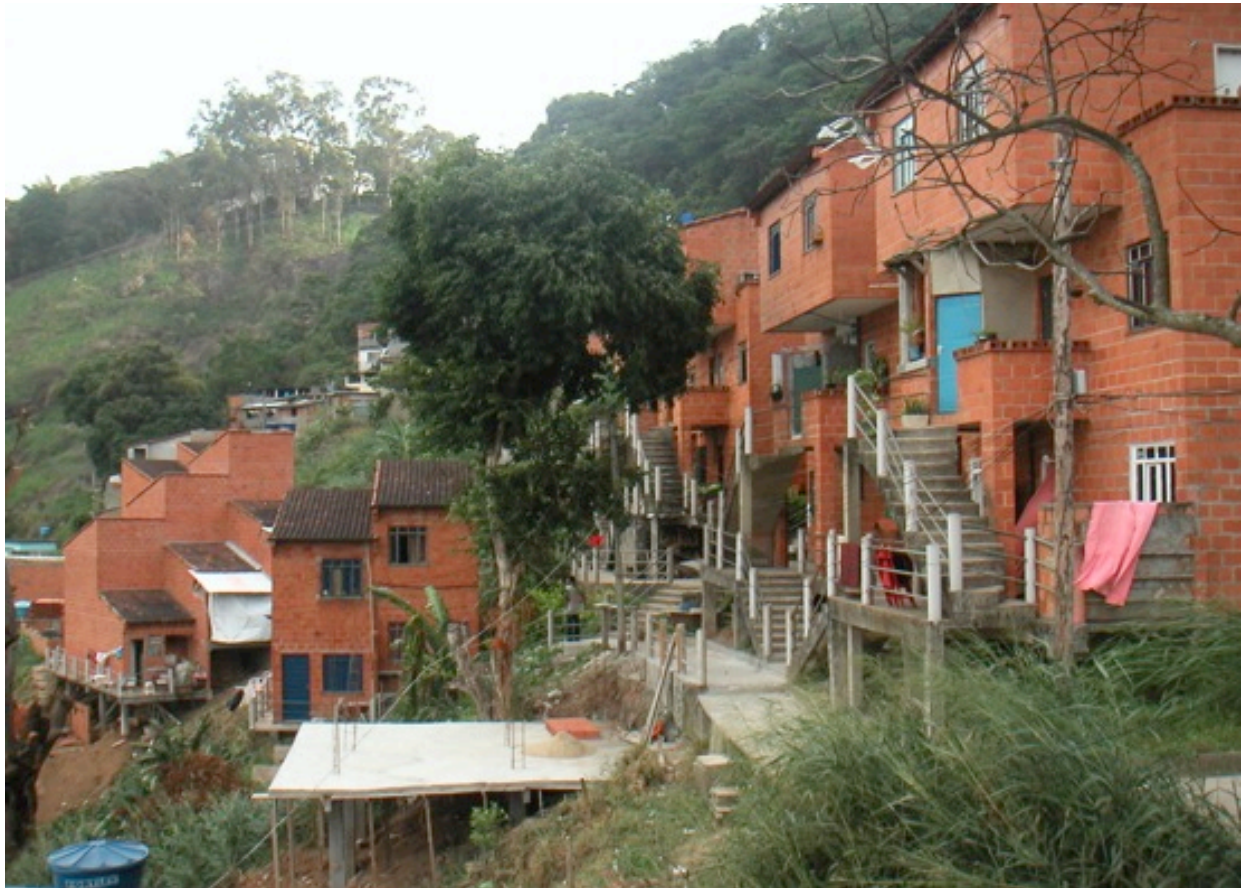
Figure 5 As casinhas, built by the Municipal Housing Secretariat under the Favela-Bairro infrastructure upgrading program from 1999 to 2001.
