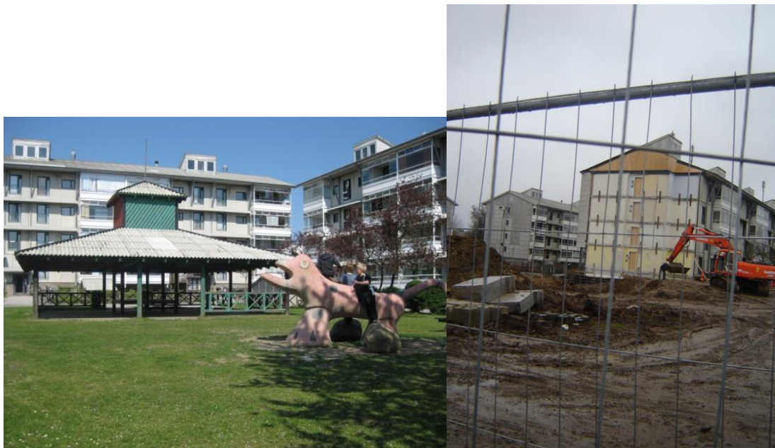
Figure 7.5 and 7.6 Dyrehaven Housing Project Demolition
