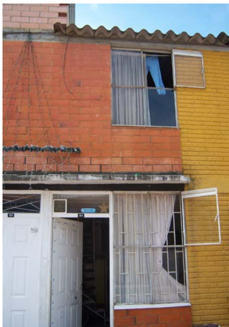
Figure 12. Exterior view of Camila's house. Source: I. Cuervo
