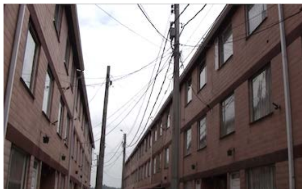
Figure 16. Main entrance alley in front of Álvaro's house showing the misplaced and dangerous electrical pole. Source: I. Cuervo
