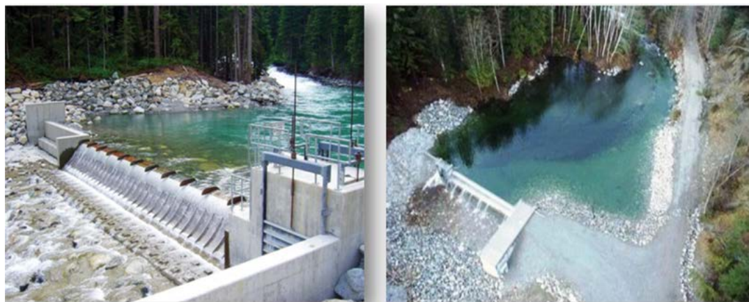
Figures 25a and b. Coanda-screen dam (weir) and view of a head pond (Courtesy of Elgin Equipment Group (EEG) (2010))
