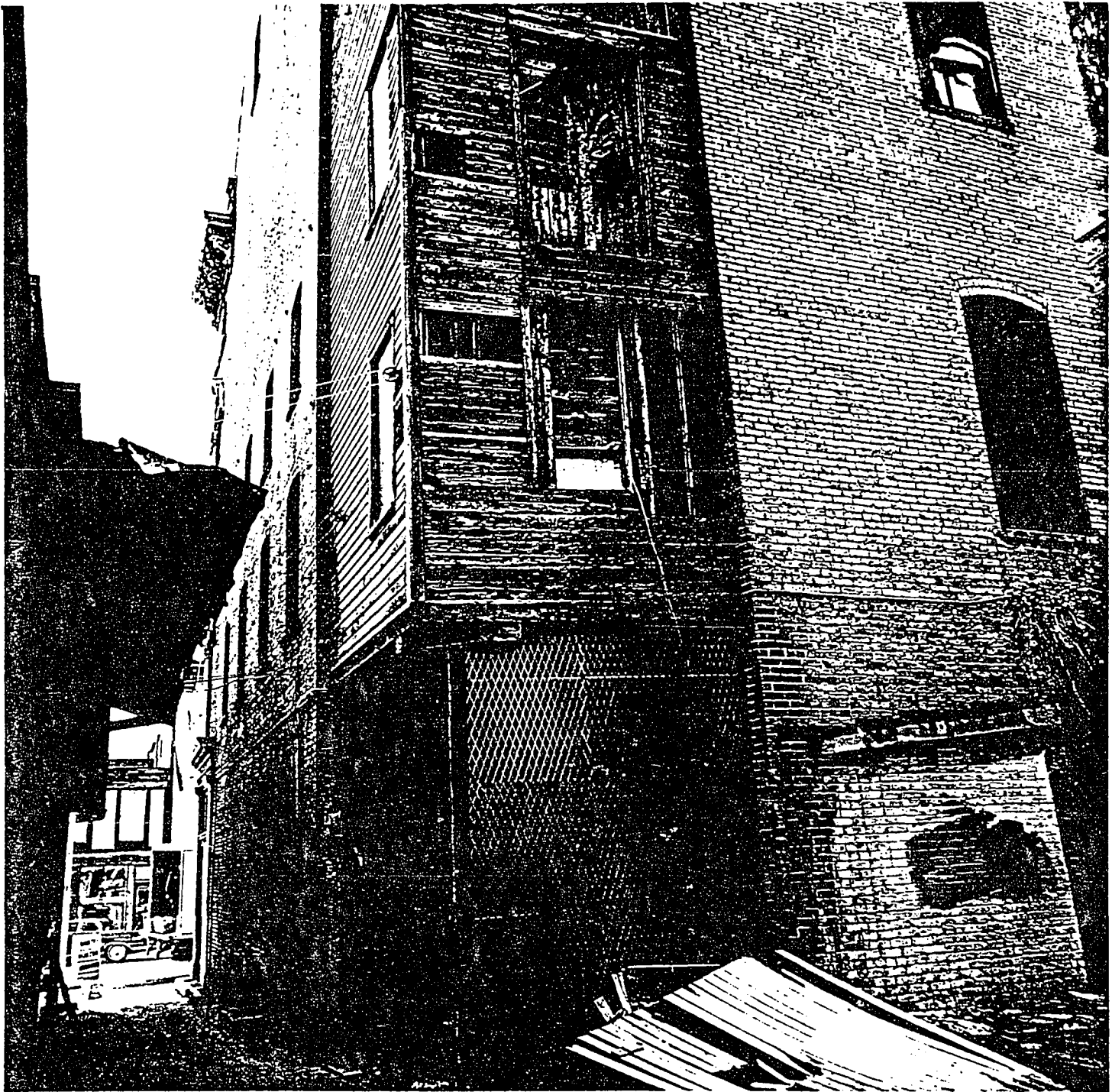
Figure 6, View of northwest corner of the building showing the alley and the external, wooden elevator housing used for the transportation of scenery.
