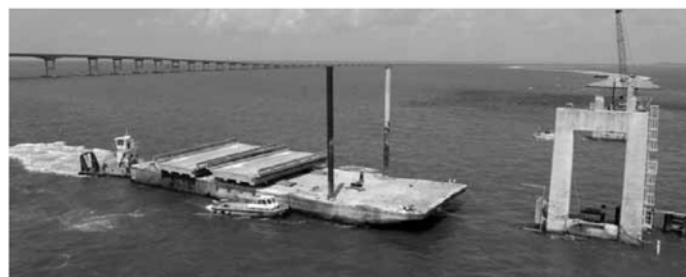
Figure 2.3 Full scale test of the barge bridge collision in Florida
