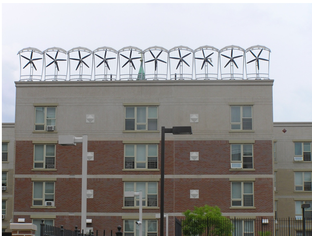
Figure 7.3 Windmills on the Roof of the Eltona (Source: Author)
