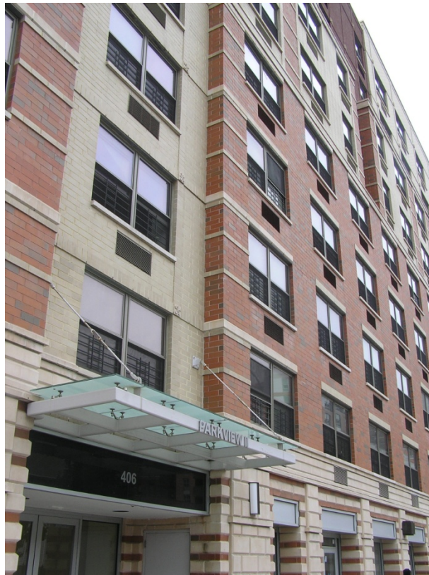
Figure 7.2 A brownfield project in Melrose Commons (Source: Author)
