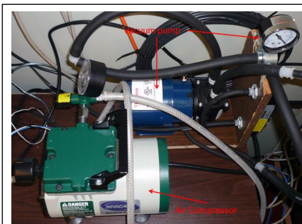
Figure 4-3: Air compressor and vacuum pump.
