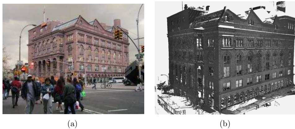
Figure 3.4: The Cooper Union building, NYC. (a) Photograph [3]. (b) 13 out of a total of 31 registered range images shown.
