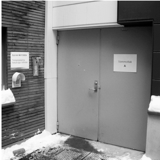
Figure 39. Service entrance that was used by all the participants that arrived from this side of the building.
