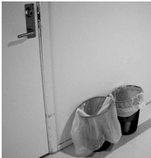
Figure 54. If the door constitutes too much of a barrier users will find ‘workarounds’ such as bins, chairs or any other objects that can keep the door open.
