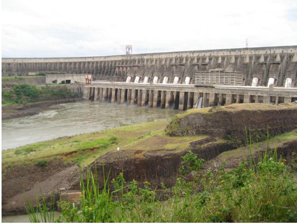
Photograph 4 Itaipú Binacional hydroelectric dam, seen from the Brazilian side. Author's photograph. April 7, 2007.
