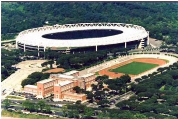
Figure 23. Rome's Olympic Stadium alongside the CONI offices and Stadio dei Marmi.
