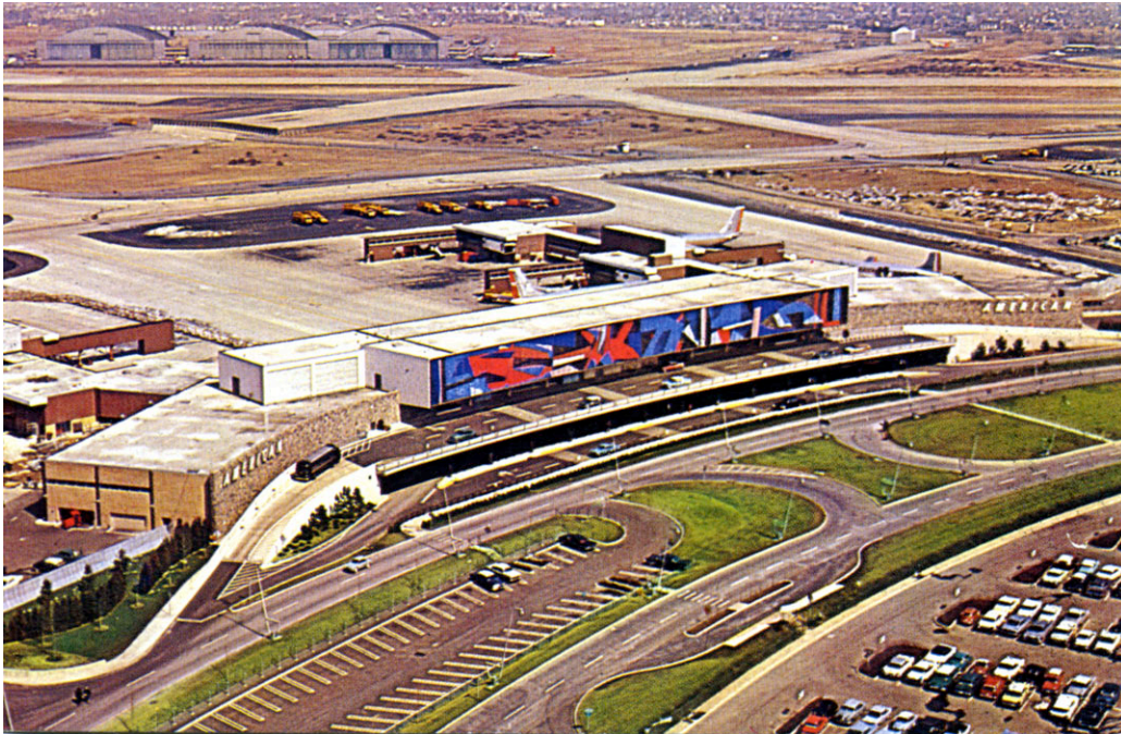
Figure 54. American Airlines Terminal, 1960, Idlewild, New York International Airport. Kahn & Jacobs, architects.
