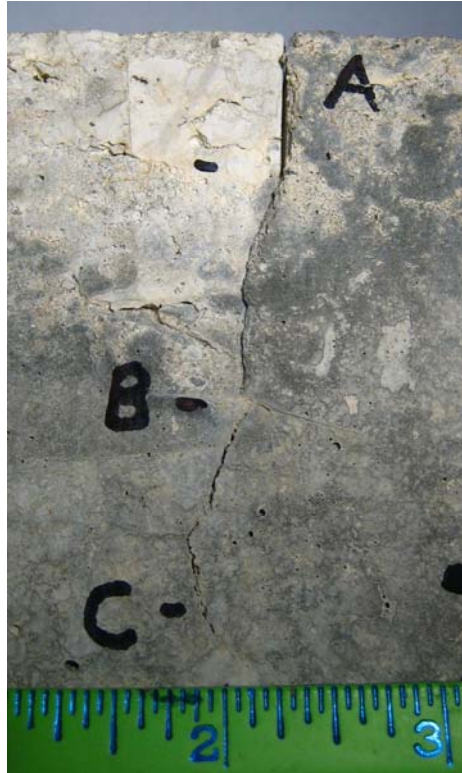
Figure 4-3: Photograph showing a closeup view of the crack originating from the plastic insert.
