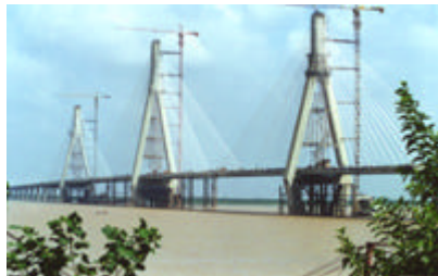
a) Dongting Lake Bridge
