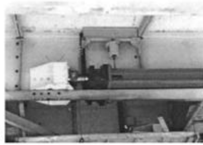
b) Variable orifice damper
