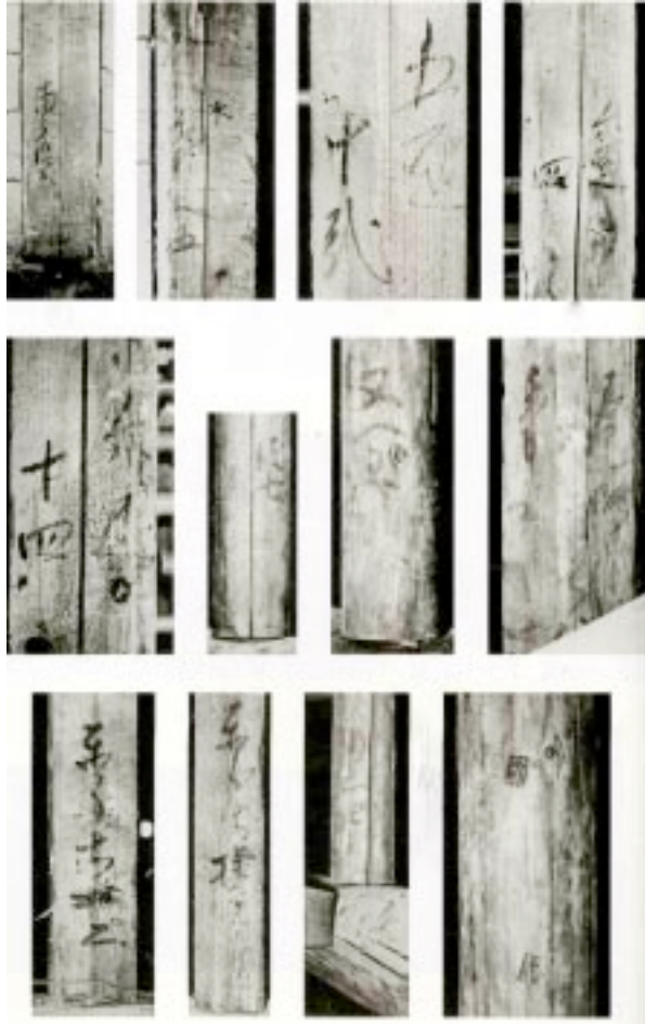
Figure 8: The Importance of a Roof. Although from the outside Shoeikan looked like a New England college building, it was built using a set of standard Japanese architectural tools, as pictures 1 and 2 show. The beams of the roof construction are connected in complex ways using many different types of joints, requiring the kind of annotation seen in picture 3. One of the main challenges of any reconstruction requiring roof removal is the procedure of dismantling that would enable it to be put back together, a painstaking process that only a handful of carpenters still know how to perform. [copyright © Dōshisha University Archives]
