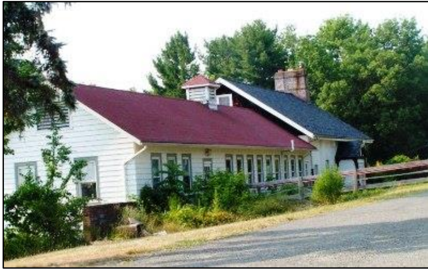
Fig. 6.4: Main building of a community program, JJC, New Jersey
