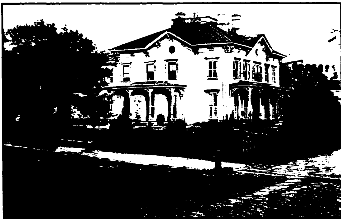
Fig. 3 Davis B. Kurtz House, Washington Street, New Castle, Pa. (demolished 1963) Photograph: Lawrence County Historical Society, New Castle, Pa.
