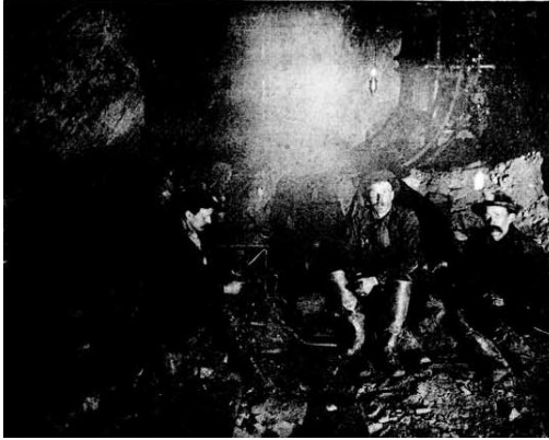
Figure 2.16: In the Tunnel Heading by Electric Light, Photograph from City of New York Aqueduct Commissioner: Report on the New Croton Aqueduct, Reservoirs, and Dams: 1883-1887 , New York City Department of Environmental Protection Archive. Courtesy of DEP Archive.
