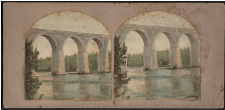
Figure 2.8: View of Section from the Lower Banks: High Bridge, New York, No. 3. : New York Stereoscopic Co. – Photographer. Created 1859-1864: Robert N. Dennis collection of stereoscopic views.
