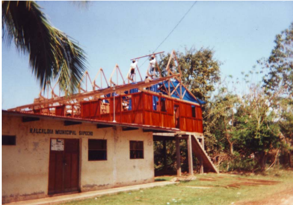
Figure 8. Community members building the Center for Community Communication in Sapecho, 2002. (Courtesy CEFREC-CAIB).
