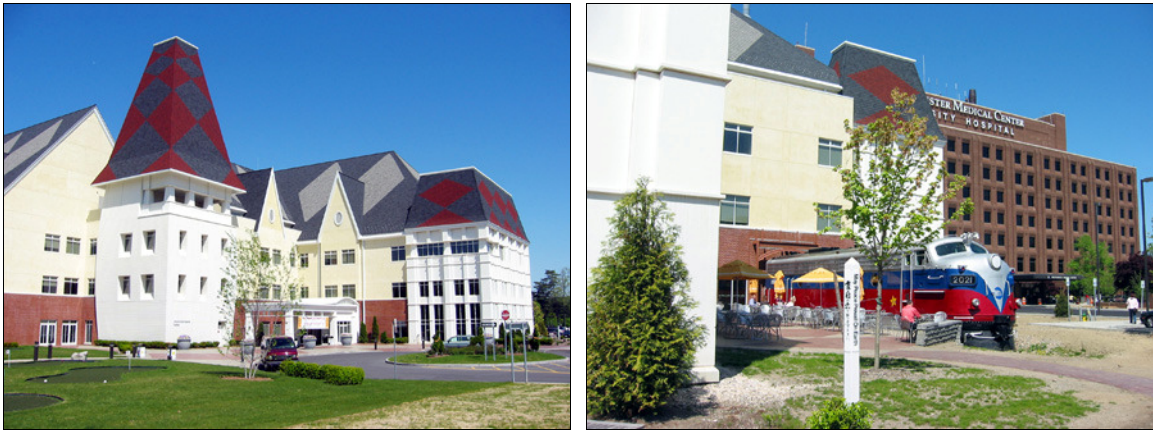
Figure 15: Images of the new Maria Fareri Children's Hospital
