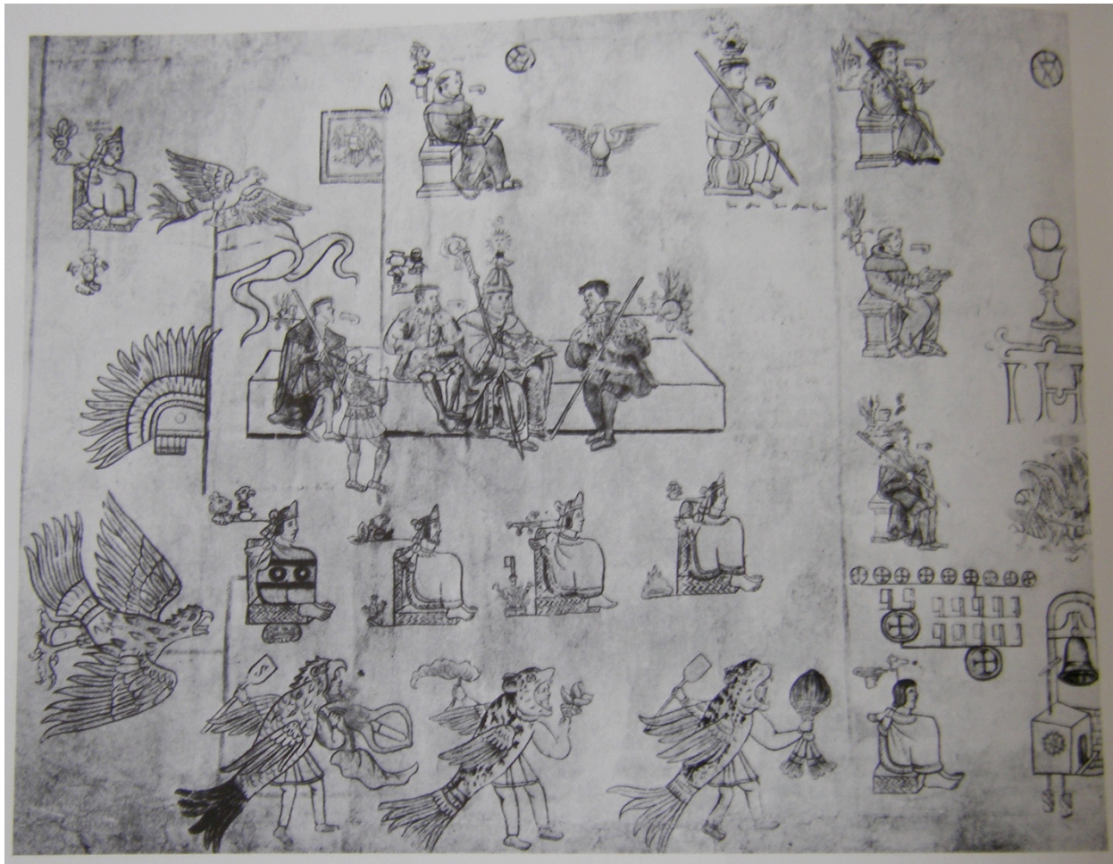
Figure 1.11 "Beginning the Construction of Mexico City Cathedral in 1562." Codex de Tlatelolco (1565). From Serge Gruzinski, Painting the Conquest: The Mexican Indians and the European Renaissance (Paris: Flammarion, 1992), 140.
