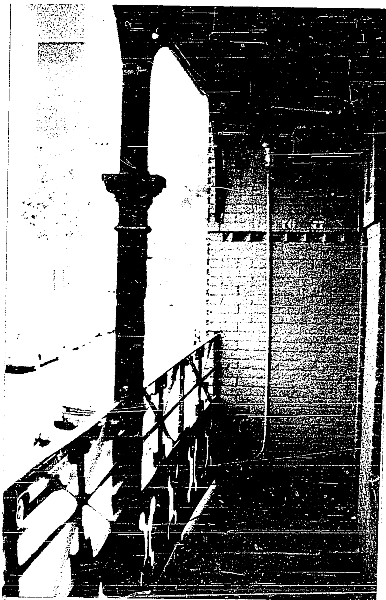
Fig. 13 Tower Buildings. View of the access balcony. Photo: Cromley.
