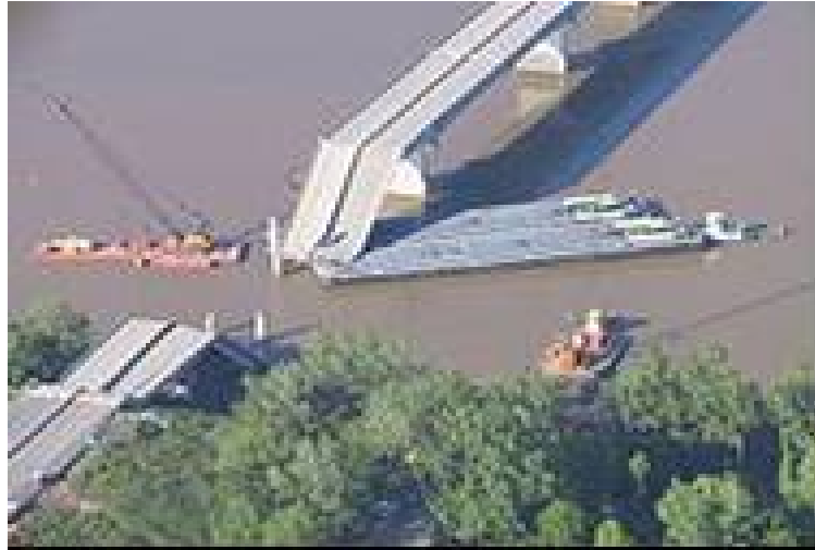
Figure 1.3 Collapse of I-40 Bridge in Oklahoma in 2002
