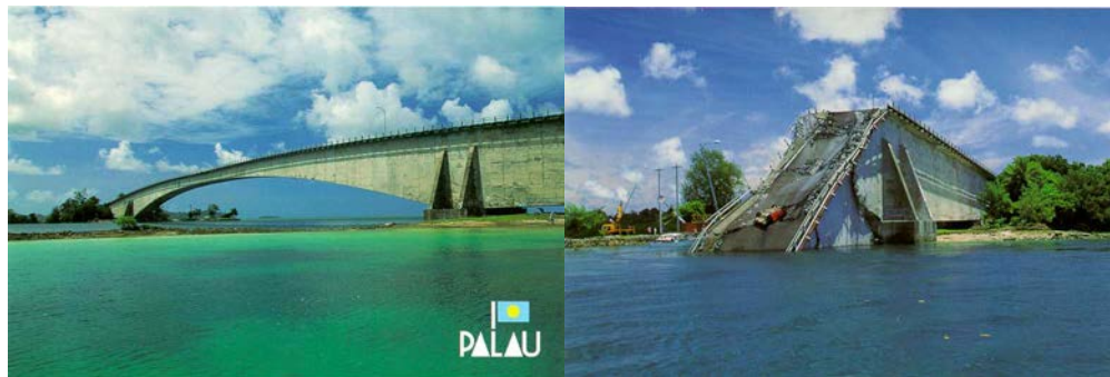
Figure 1.5 Collapse of the Koror-Babeldaob Bridge in 1996
