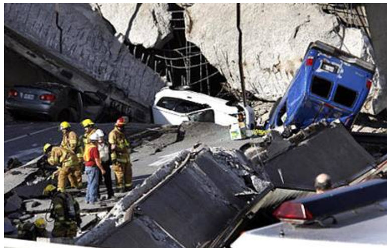
Figure 1.4 Collapse of Highway 19 Overpass, Laval Quebec (2006)
