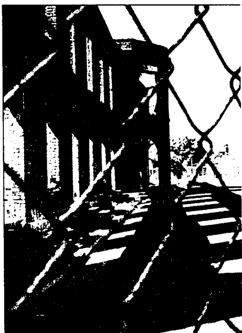
Figure 1.12: Burnt out shell of the Old Courthouse – once housing the Town’s Hall, now sits behind a 10 ft. chain link fence on the square.
