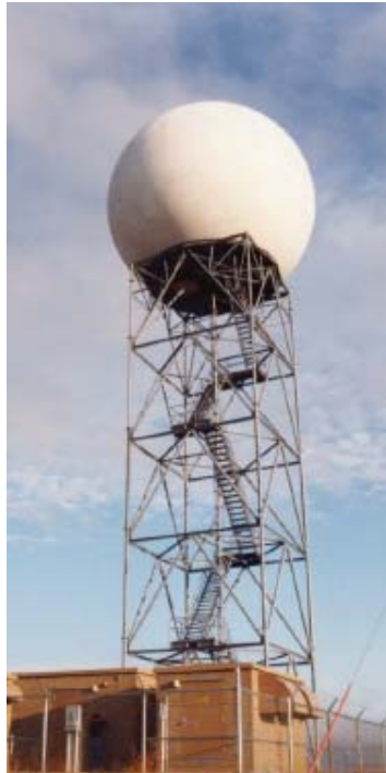
Figure 3: WSR-88D radar antenna
